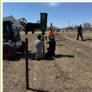
Volunteers building the track
